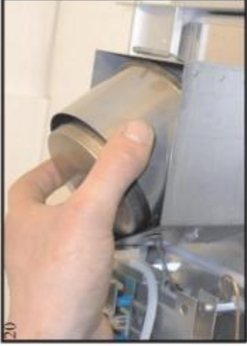
Remove the burner by tilting it as shown.
