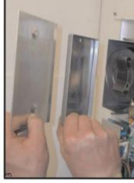
Remove the burner heat shield and then the bottom lock plate.
